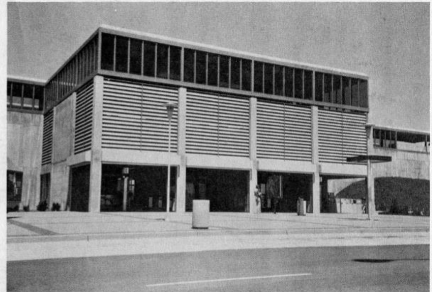
(b) CENTRAL PORTION OF BUILDING
